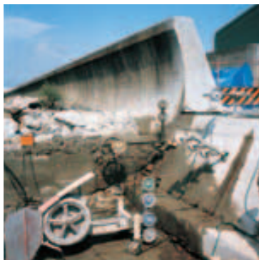
Diamond wire saws at work
